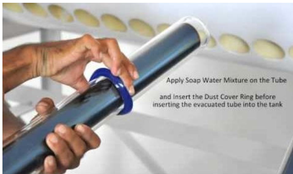
Figure 118 Assembly of evacuated tube with storage tank
