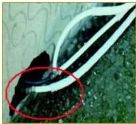
Figure 10: Rising waterproofing damaged by piping passage / Waterproofing roof damaged by steel structure
