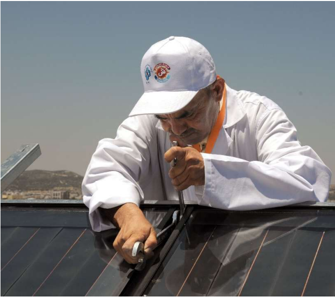
Tightening by key and against key the top and bottom collector series connection
