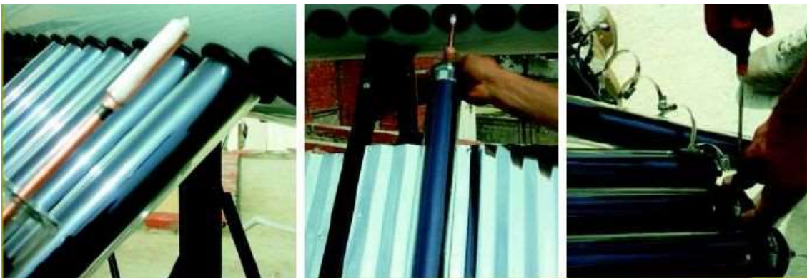
Fixing up vacuum tubes in manifold inside the tank/ Fixing bottom tubes in aluminum slide
