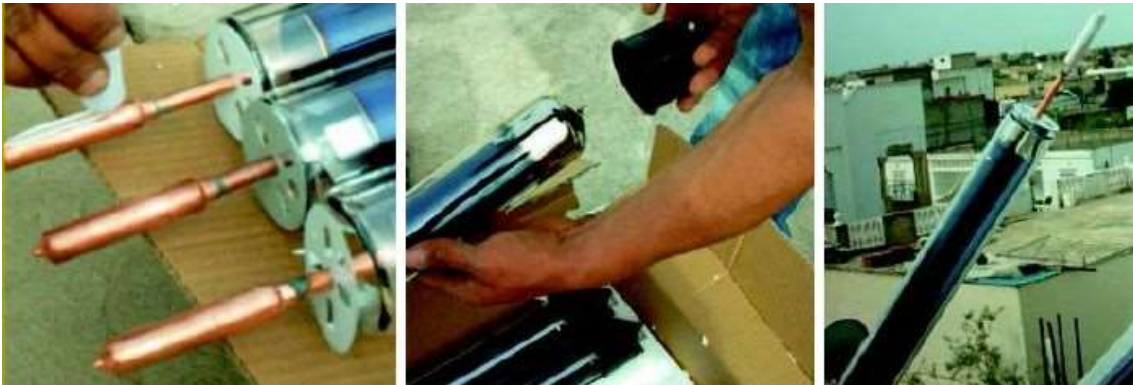
Preparation of vacuum tubes for mounting/application of thermal paste/ fitting of UV Rubber cap
