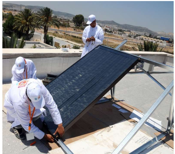
Fixing collector on bottom and top track
