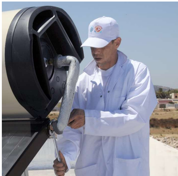
Connection and tightening of the Collector-Tank hot water piping. It should be insulated by "Armaflex" and protected from the UV from the sun
