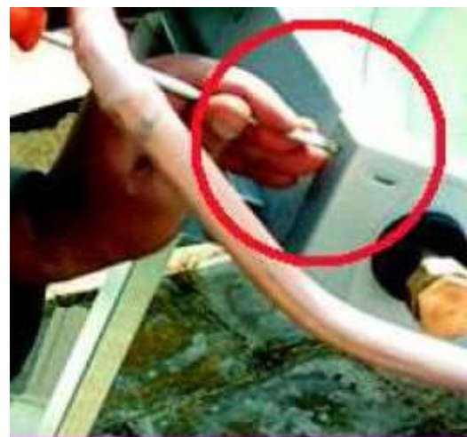
Collector orifice drain control
