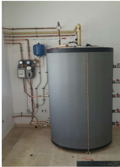
Figure 21: Storage tank location for forced system
