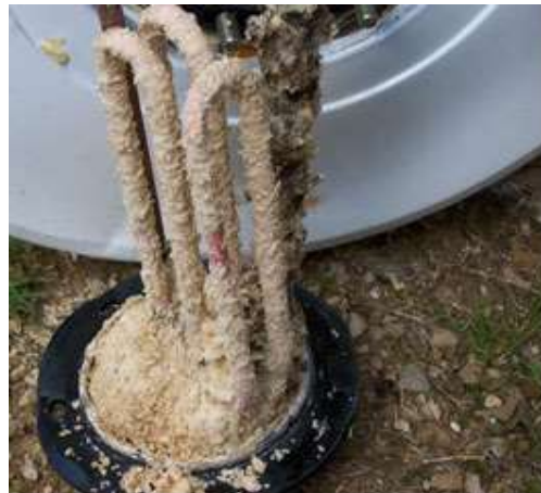
Figure 40: Electric back up covered by the limestone
