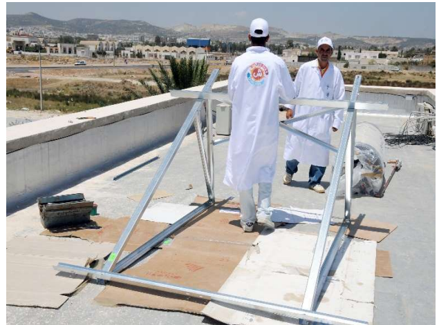
Structure reinforcement by X back arrangement / Fixing Track collector on triangular steel structure
