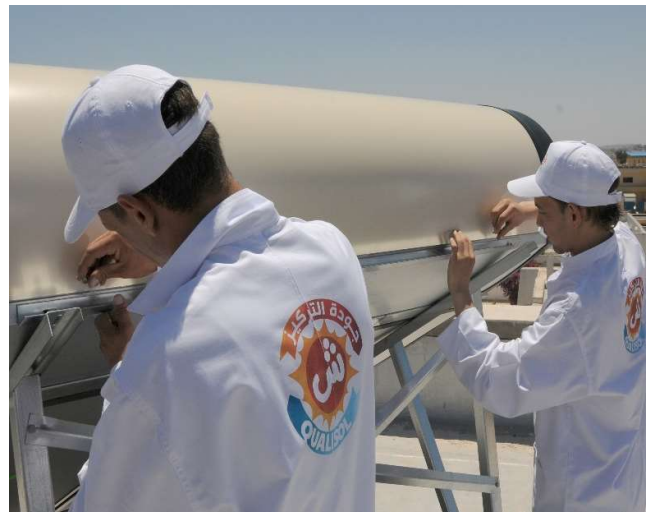
Fixing tank on the frame
