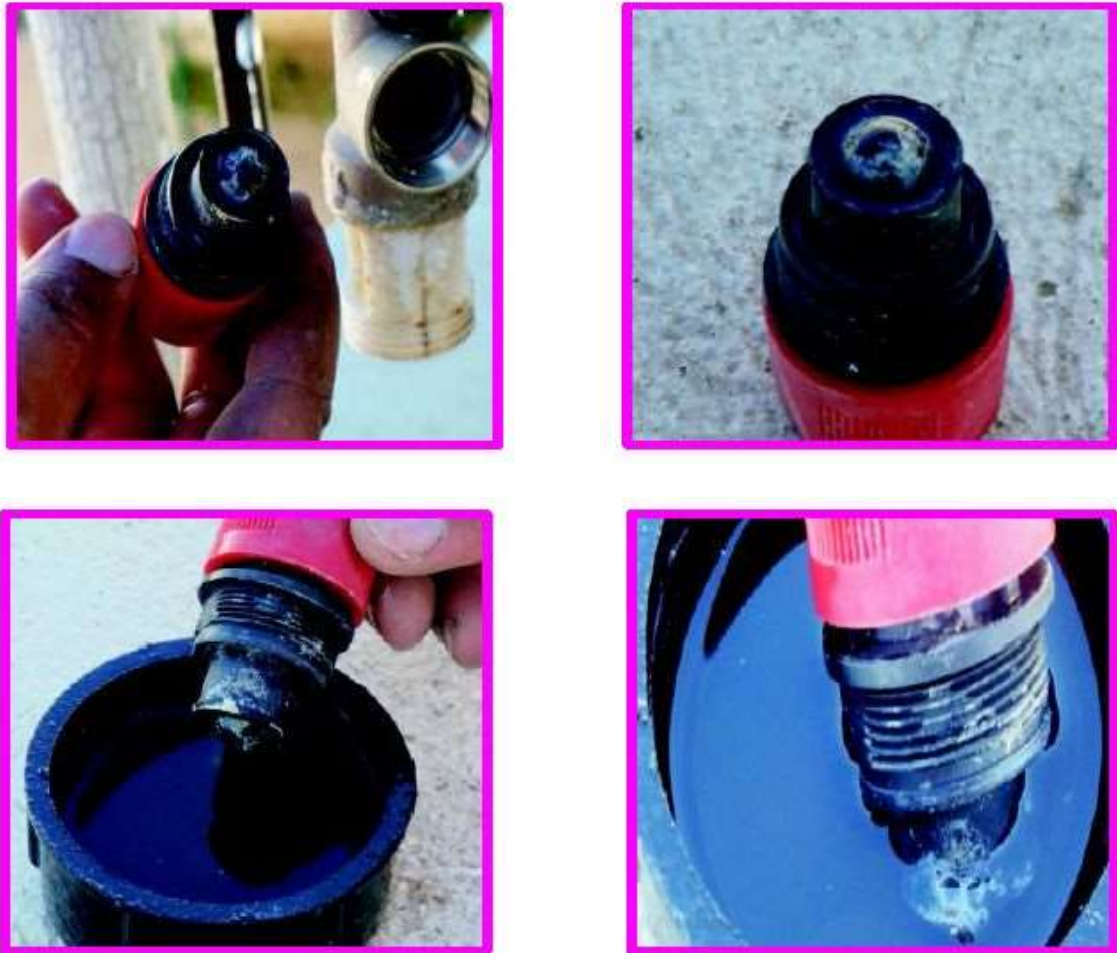
Figure 35: Descaling the non-return safety valve mechanism steps
