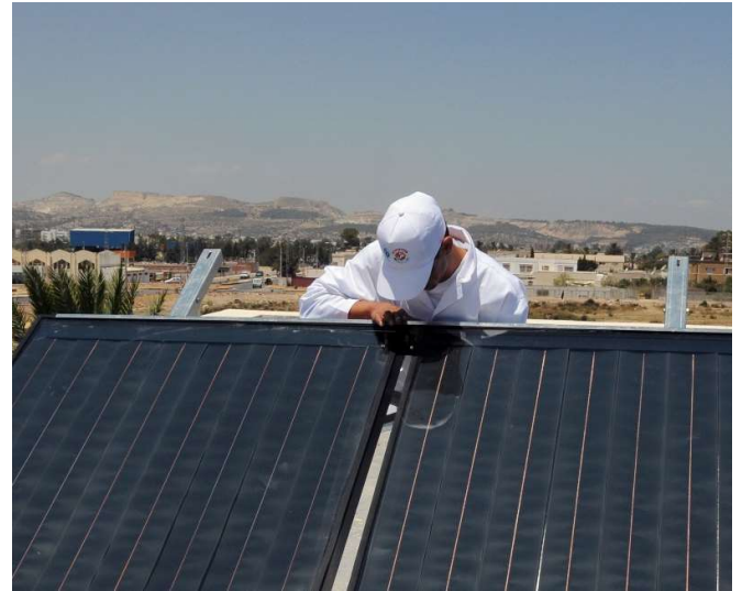
Tight the fixation on top track
