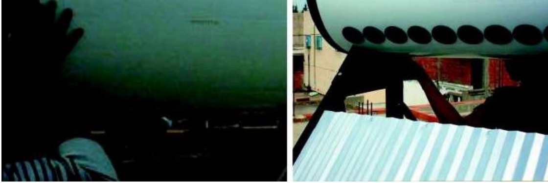
Tank mounting and fixation
