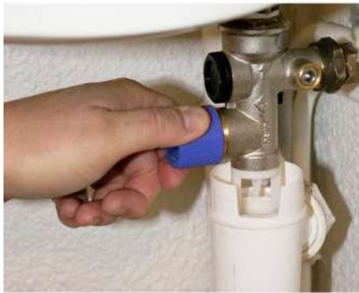
Figure 31: Purge button operation
