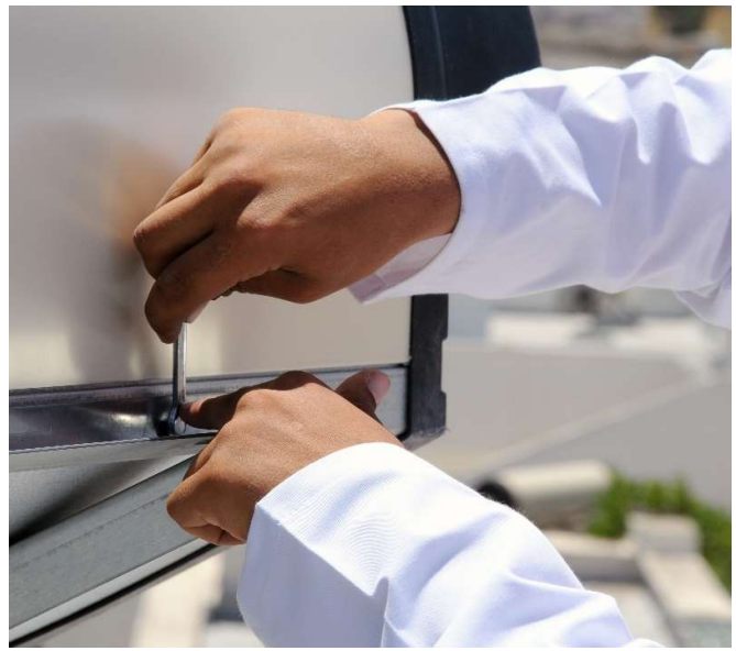
Tightening tank fixation
