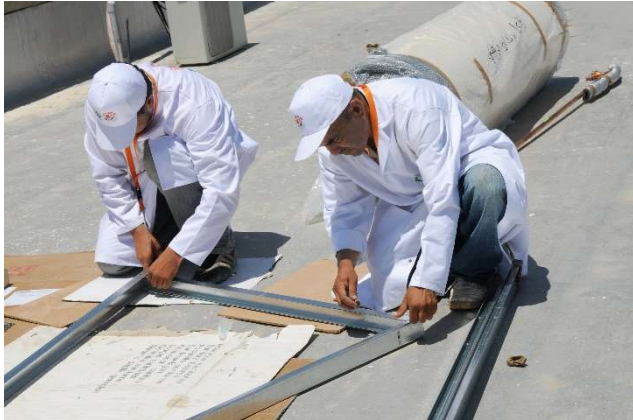
Steel structure is assembled on the floor
