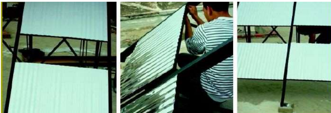
Fixing the reflectors on the steel structure
