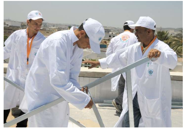
Lateral triangular steel structure are assembled on the floor
