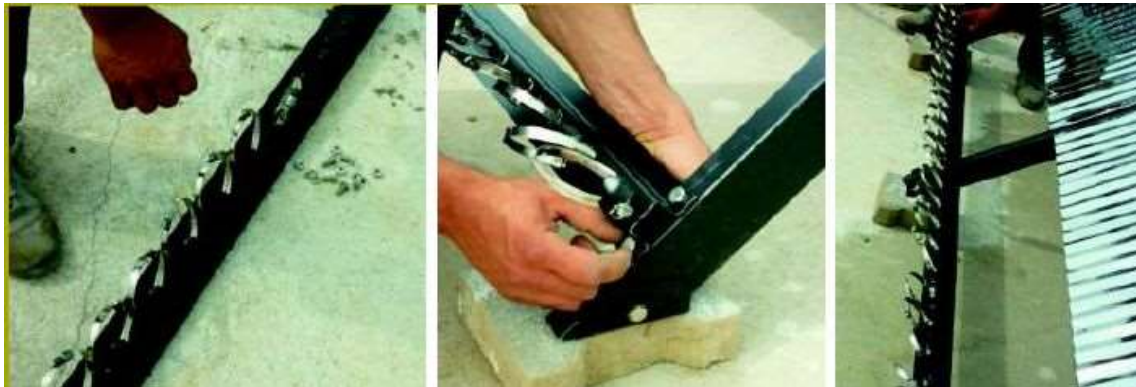
Fixing collars insertion
