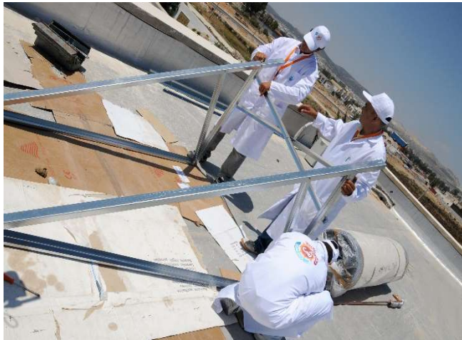
Structure reinforcement by X back arrangement / Fixing Track collector on triangular steel structure
