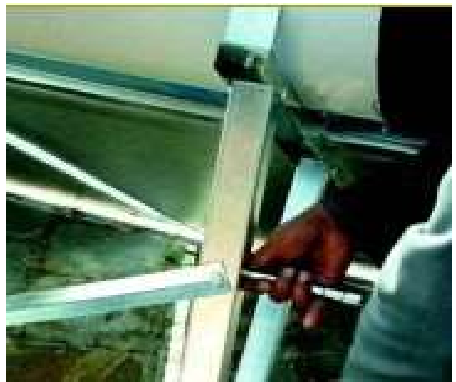
Tightening the X back fixation after tank mounting
