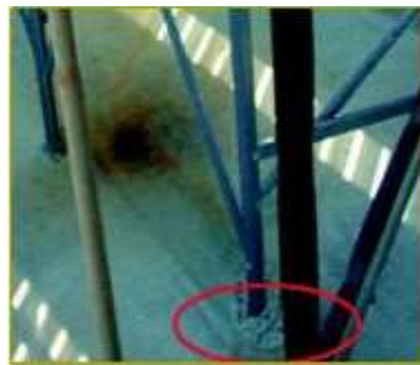
Figure 10: Rising waterproofing damaged by piping passage / Waterproofing roof damaged by steel structure
