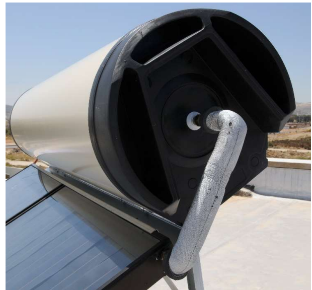
Connection and tightening of the Collector-Tank hot water piping. It should be insulated by "Armaflex" and protected from the UV from the sun
