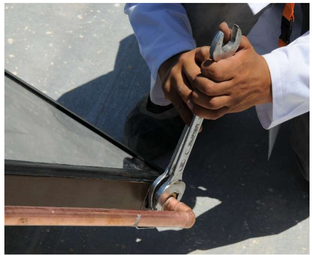
Connection and tightening of the Collector-Tank cold-water piping
