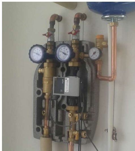
Figure 22: Example of pump station mounting onto wall
