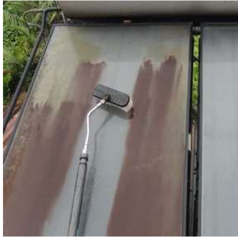
Figure 29: Cleaning dust from dirty Collector Surface
