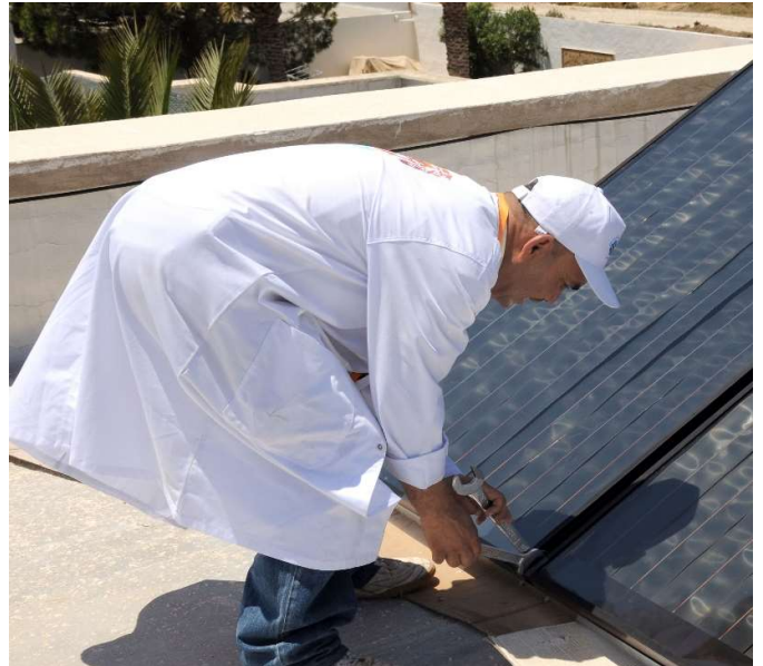
Tightening by key and against key the top and bottom collector series connection
