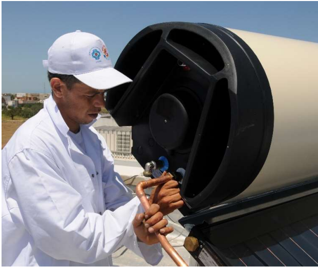
Connection and tightening of the Collector-Tank cold-water piping
