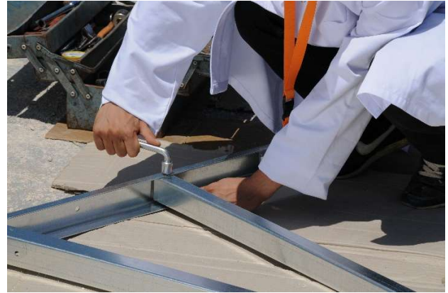
Steel structure is assembled on the floor
