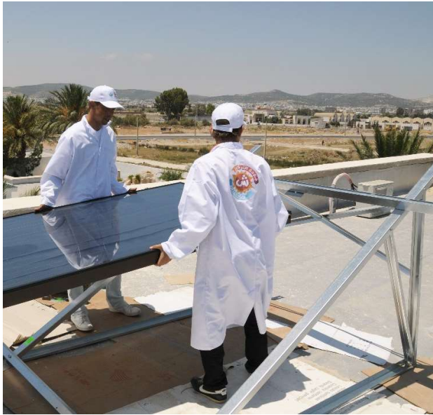
Fixing and positioning the frame
