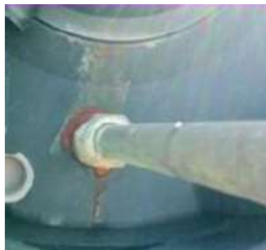
Figure 38: Tank leaking
