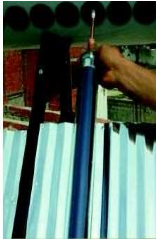
Fixing up vacuum tubes in manifold inside the tank
