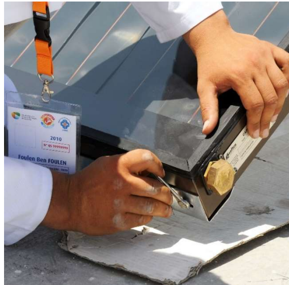
Fixing collector at frame bottom
