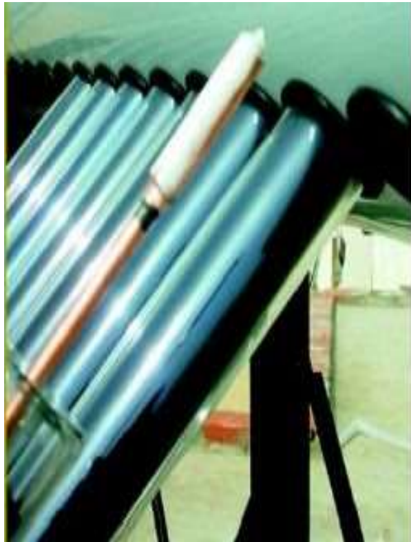
Fixing up vacuum tubes in manifold inside the tank
