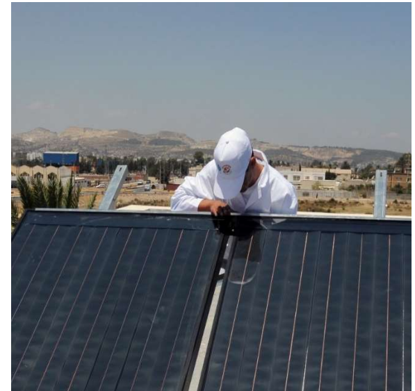
Fixing collector at frame top
