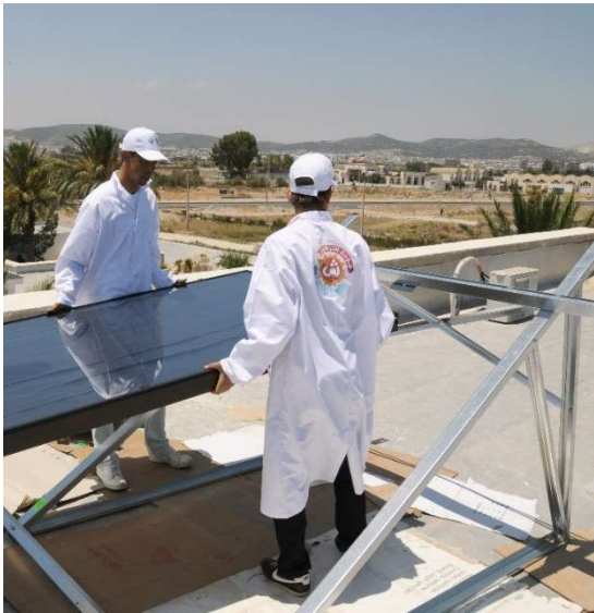
Fixing and positioning collector on the frame
