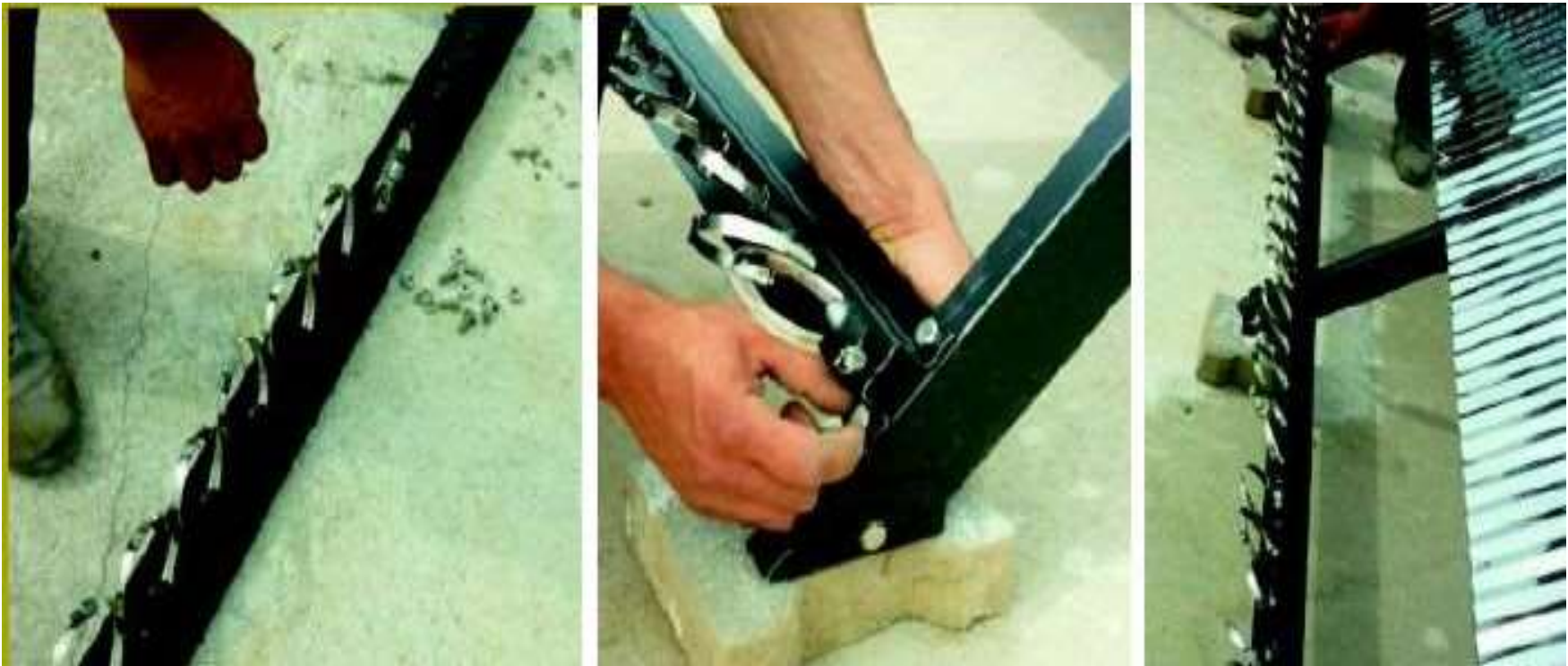
Fixing collars insertion on frame support
